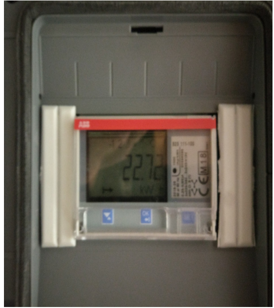
Photo 9: Installation of energy meters
