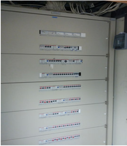
Photo 8: Modification of power lines for lighting fixtures
