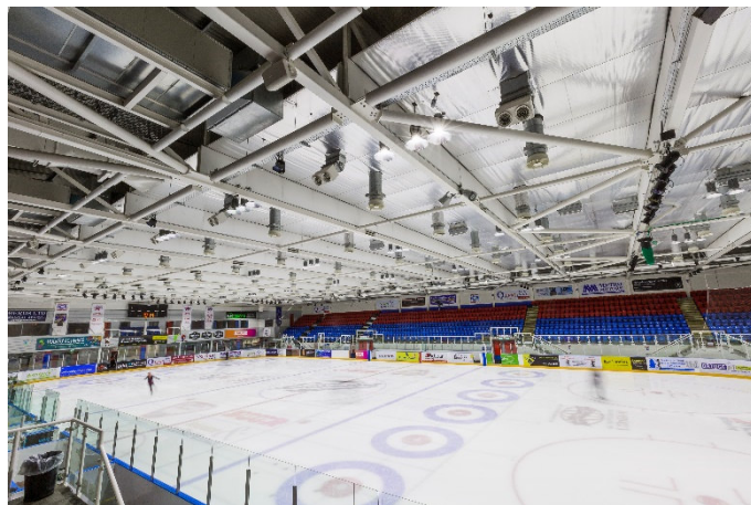
Photo. New LED lighting at Dundee Ice Arena
