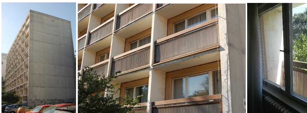
Picture 1 ŠD5 before renovation
