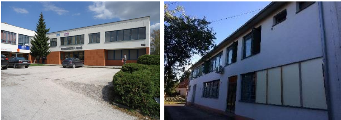
Picture 2 Service centre before renovation
