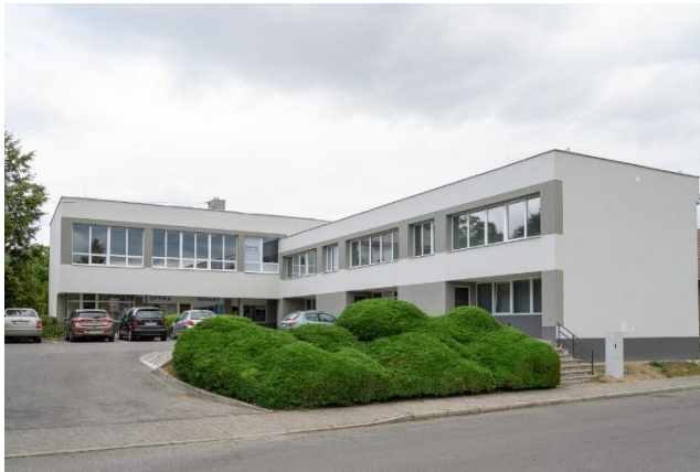
Picture 3 Service centre after renovation
