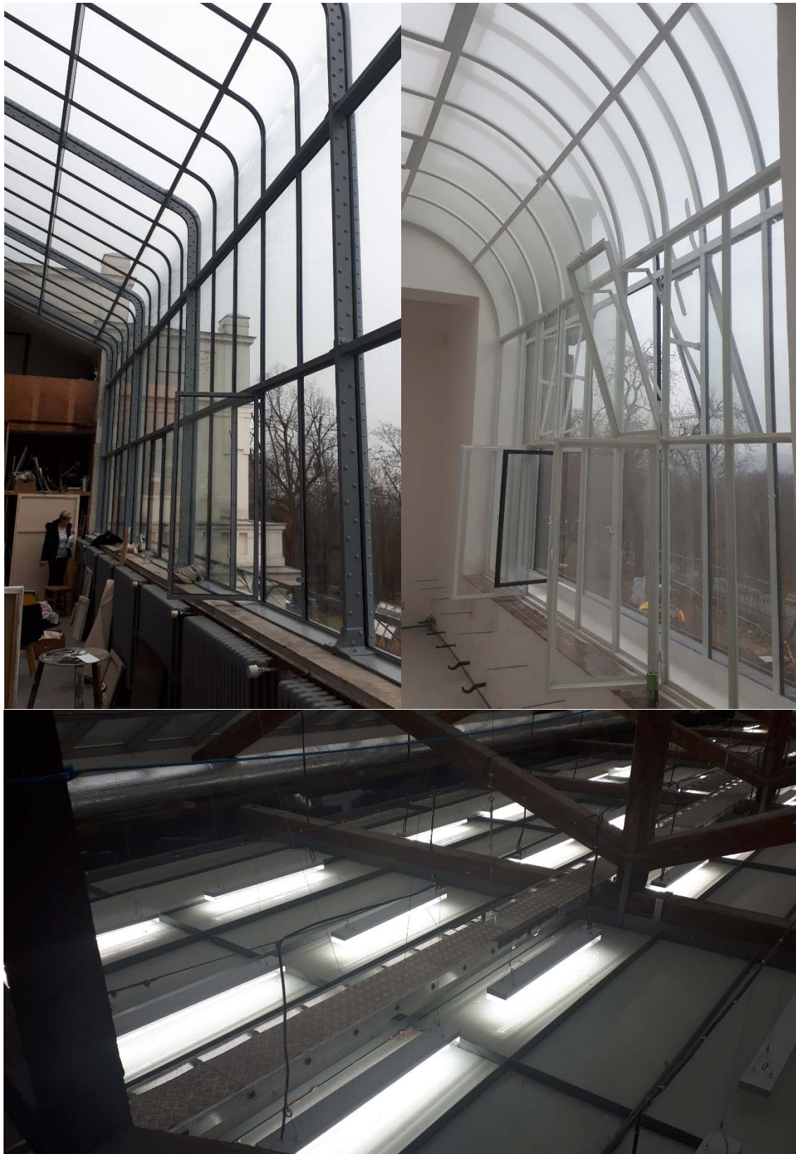
Figure 1 Photos of installed measures
