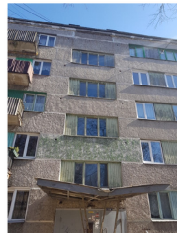
Old wooden windows and wood-beaming frames
