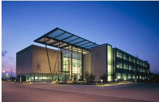
PV car ports, EV charging, ground source heat pump & various efficiency measures for municipal offices in Cambridgeshire, UK
