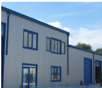
Efficient refrigeration a distributional centre Ruvela, Sofia
