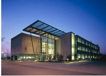
PV car ports, EV charging, ground source heat pump & various efficiency measures for municipal offices in Cambridgeshire
