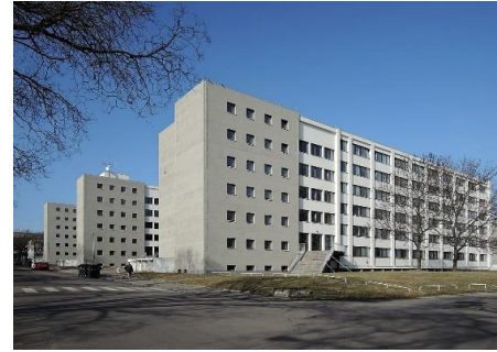
Dormitory building complexes of Czech Technical University in Prague
