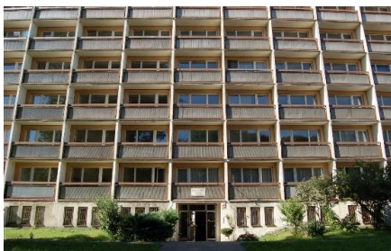
Deep retrofit of student dormitory ŠD5 - Starohájska 2900/8 in Bratislava
