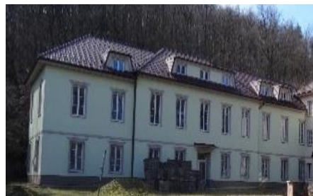
New heating management system implementation in Psychiatric Hospital of P. Pinel
