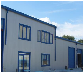
Efficient refrigeration at distributional centre Ruvela, Sofia
