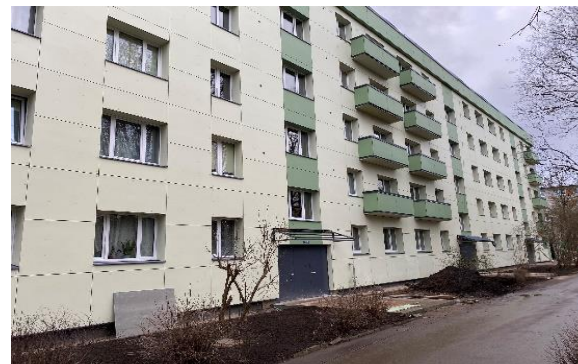
Deep retrofit of residential building in Riga
