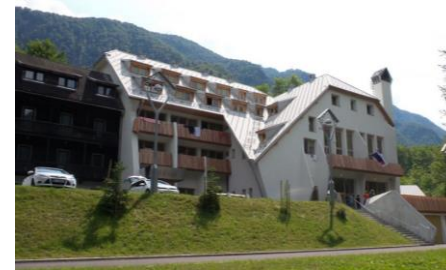
Centre for School and Outdoor Education (CŠOD), Bohinj
