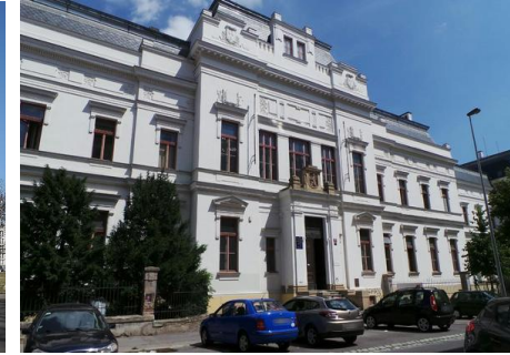
Retrofit of 11 000 m 2 buildings of Academy of Fine Arts in Prague
