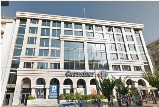
Energy upgrade of the heating and cooling system for 1 792 m 2 big office building in Athens.
