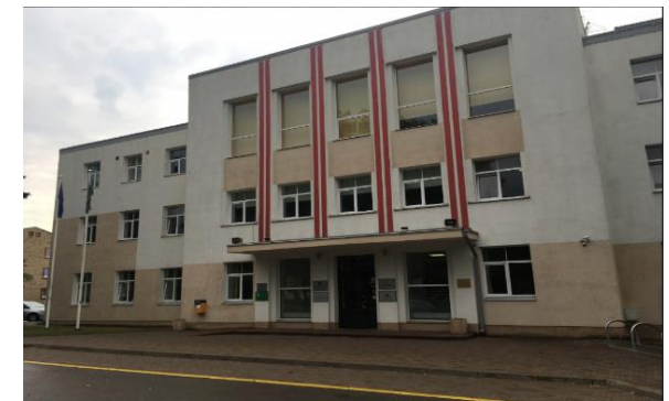
PV for Gulbene municipality office building
